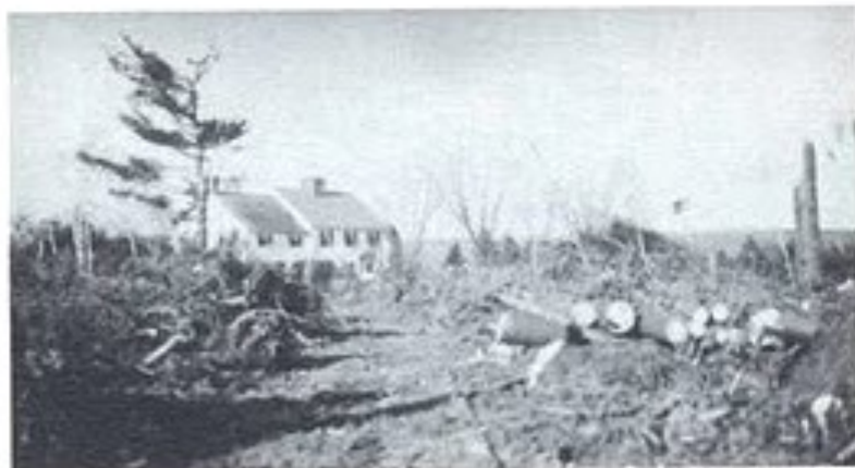
Hurricane damage in grove by house 1918
