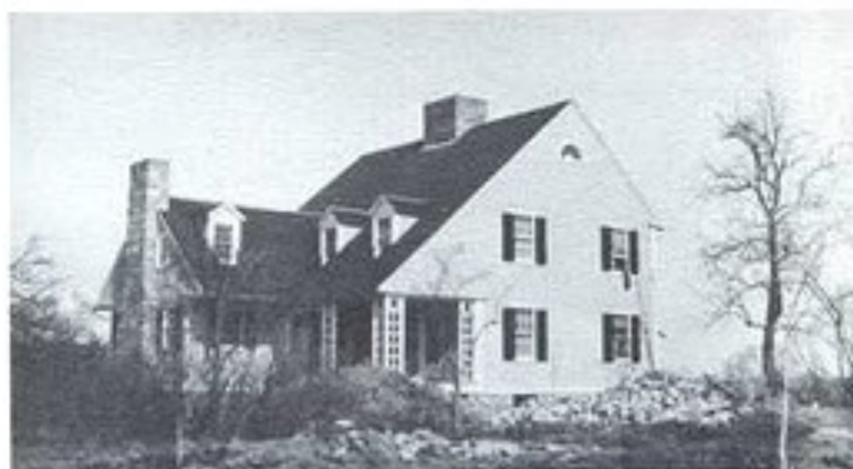
Farmhouse in course of construction—Year 1915
