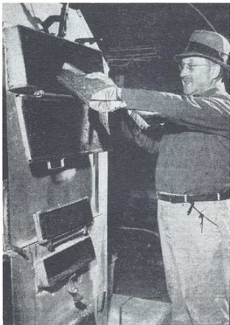
Wood-burning furnace with Manager Edion Stocking putting in soft wood slabs. It was found that this temperature-controlled unit which is stoked only once or twice a day, can heat 12 rooms and 2 baths on $62.50 worth of wood a year.
