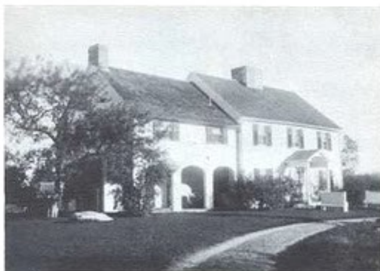
Addition to Farmhouse 1924
